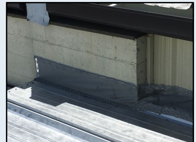
Add Dek-Strip to stop leaks between two buildings
