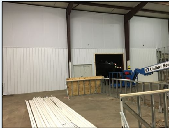
Liner Panels Walls &/Or Ceiling
