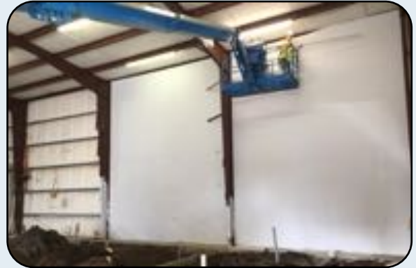
Low-E Insulation Walls &/Or Ceiling
