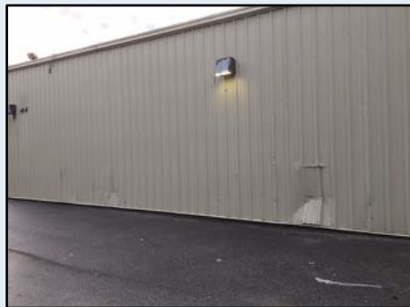
Repair damaged wall panels with new panels
