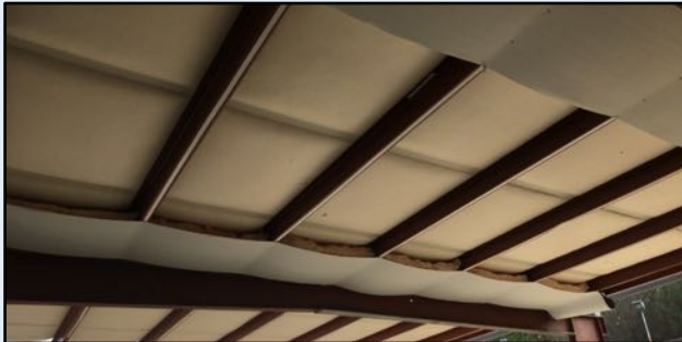
Low-E Insulation Walls &/Or Ceiling
