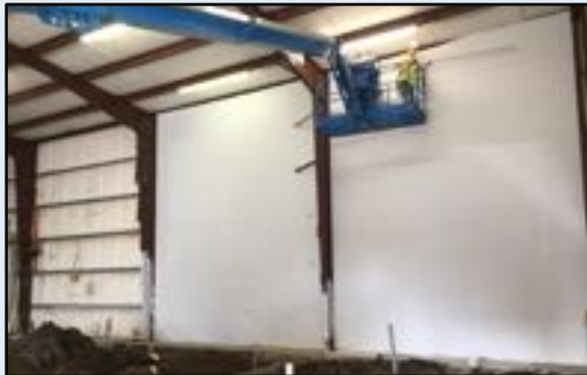
Interior Insulation Before & After
