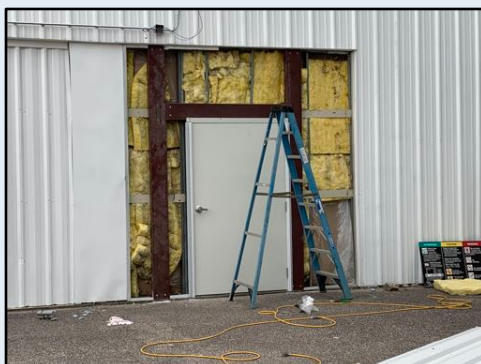
Add a framed opening with walk door in a metal building
