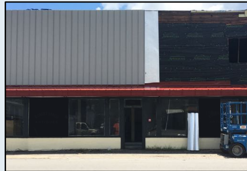
Wall Panels Before & After
