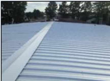
Replace Roof Panels
